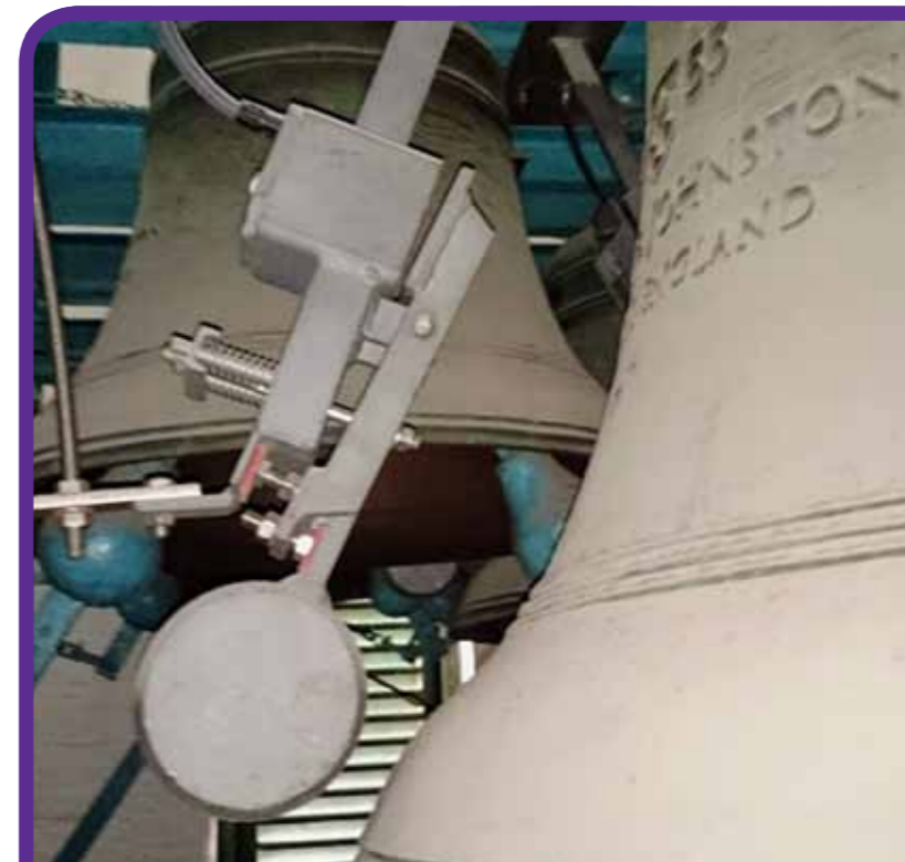
PHOTO 6 — Bell striking hammer mechanism for No. 7 Bell
