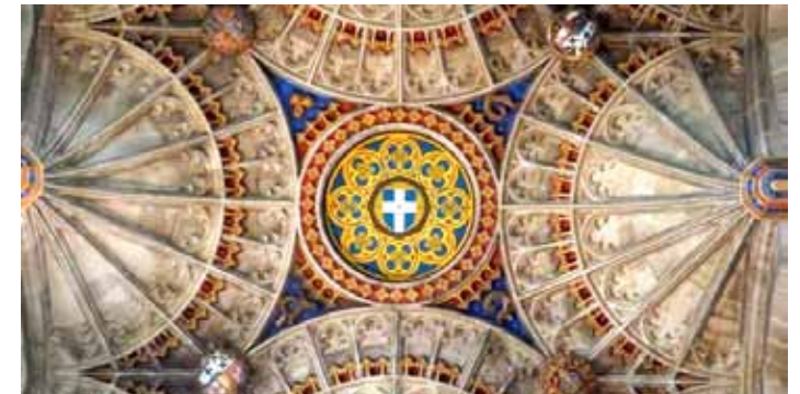
Interior of the Harry Bell Tower, Canterbury Cathedral
